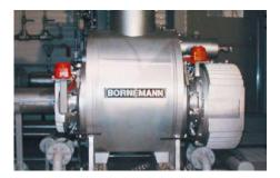
CNRL in the Cold Lake region in Canada uses over 140 pumps with approximately 500 EagleBurgmann **HSHJ92S1/80-E3** seals. The seals are fitted in Bornemann twin screw multiphase pumps. Operating conditions: Gas content ... 95 %; p ... 6 bar (87 PSI); t = 150 °C (302 °F); n = 1,200 min<sup>-1</sup>.
