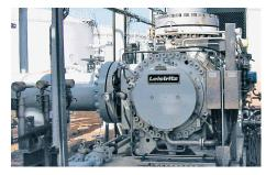
In a pump station operated by Exxon Mobil in Africa, our **SHV-D4/170-E1** (API Plan 54) functions as a dual seal for a twin screw multiphase pump from Leistritz. Operating conditions: Gas content ... 99 %; p = 60 bar (870 PSI); t = 54 °C (129 °F); n = 1,200 min<sup>-1</sup>.
