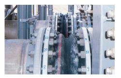
In the Middle East, oil rigs and ships are equipped with safety hoods of type **MA-1** as fire-protection devices for rubber expansion joints used in the fire-extinguishing system and in pipelines to pump flammable liquids. The hoods have been certified for marine applications by Bureau Veritas.
