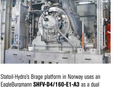
seal in an Aker-Kvaerner water injection pump.
