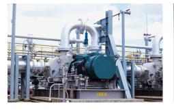
EagleBurgmann provided mechanical seals and a retrofitting concept for Petropiar/Ameriven (PDVSA Chevron Texaco) in Venezuela. The crude oil is now reliably sealed in a twin screw pump from Bornemann Pumps using an **HSHJ47GS6/140-E1**, despite the high viscosity. Operating conditions: p ... 50 bar (725 PSI); t ... 60 °C (140 °F); n = 1,185 min<sup>-1</sup>.
