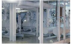
In Western Siberia, Rosneft relies on an EagleBurgmann cartridge **SH6/125-EF1** (API Plan 32) single seal to seal a Rosscor twin screw multiphase pump. Operating conditions: Gas content ... 97 %; p ... 40 bar
