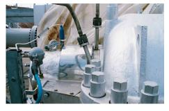
BTC (Baku-Tbilissi-Ceyhan) in Turkey has applied EagleBurgmann **SHF3-D/135-E1** dual seals and the **SHV-D3/170-E1** in the crude oil pipeline pumps provided by Ruhrpumpen GmbH. Operating conditions: p = 1 bar (15 PSI); t = 5 °C ... 40 °C (41 °F ... 104 °F); n = 1,490 min<sup>-1</sup>; p = 74 bar (1,073 PSI); t = 30 °C (86 °F); n = 1,800 min<sup>-1</sup>.
